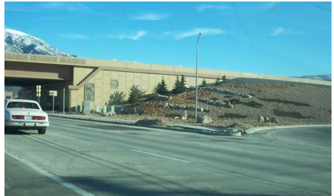
Picture 5 – An example of both water wise landscaping and bridge enhancements.
