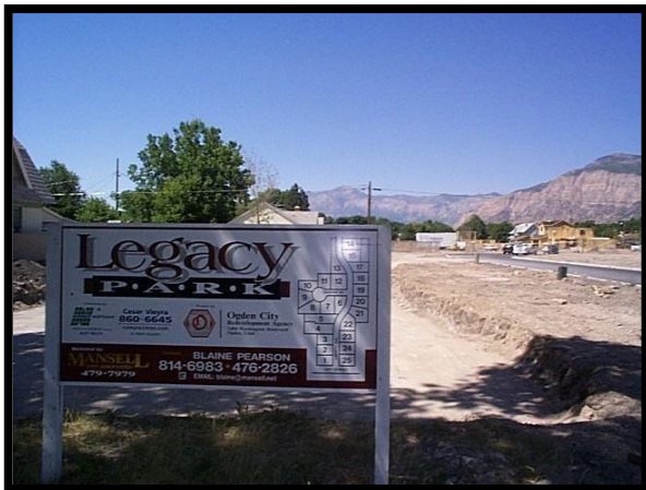
Figure 7.3 -Construction on the Legacy Park subdivision on 24 th Street
